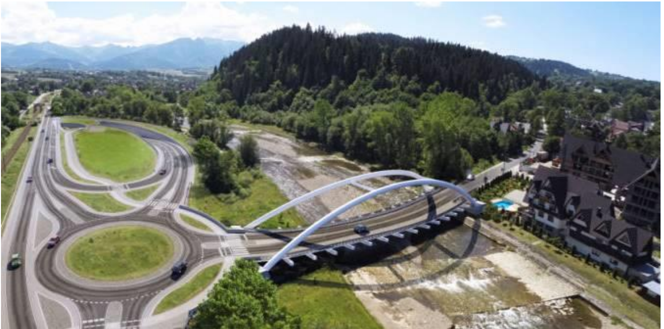
Poronin Bridge (Poronin), M48/M56 DST520 Carbon Steel, 2018
