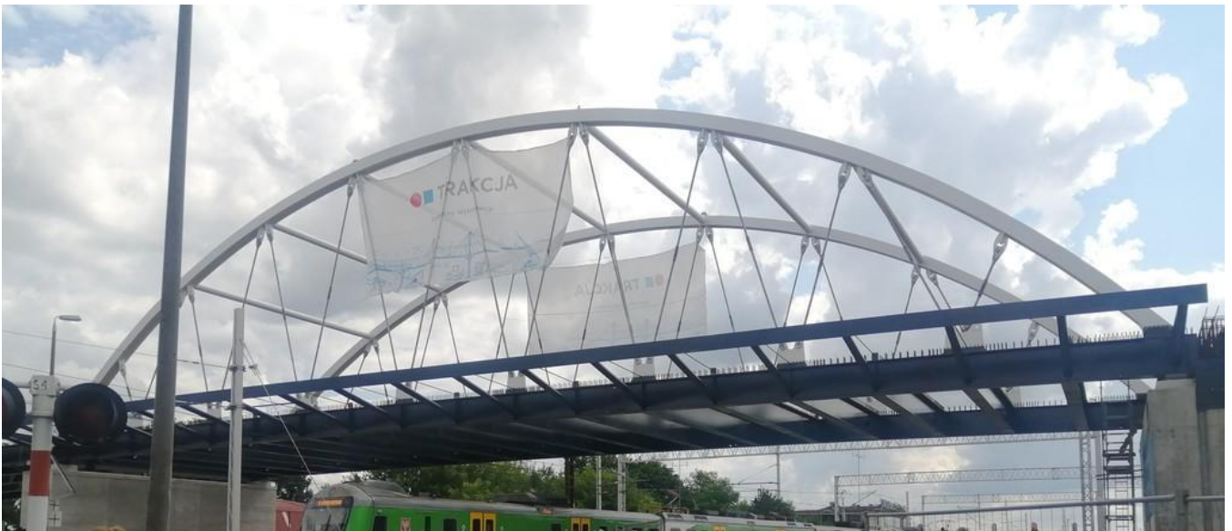
Lowicz (Poland), DST520 M76, 2020 Span length: 43m.
